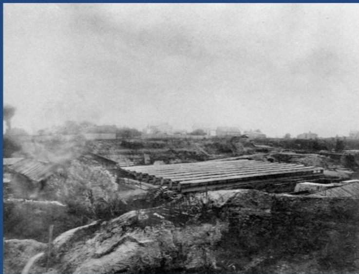
Bricks drying on racks in Ramsden Park (1880s)
