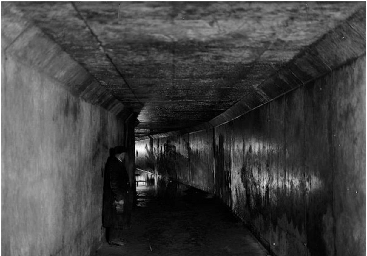
February 16, Rosedale Creek Sewer east from Sta 632 1931 - Rosedale Creek Sewer near Ramsden Park City of Toronto Archives Fonds 1231, f1231_it1293
